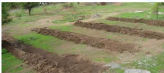
Figure 3: Continuous Contour Trenches
