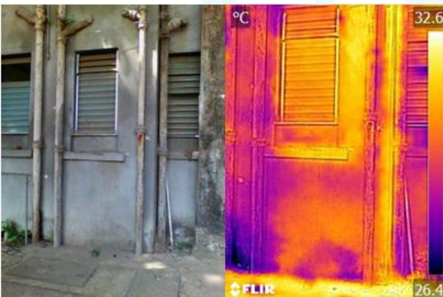
Figure 6: Behind Computer Department Toilet
