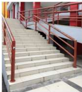
Figure 7: Tri Lomba Juang Stair
