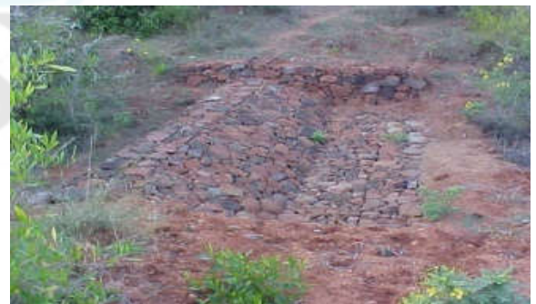
Figure 3.5 (a) Rock fill-dam
