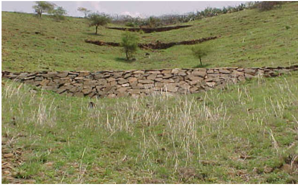
Figure 3.5 (b): Loose Boulder Structure
