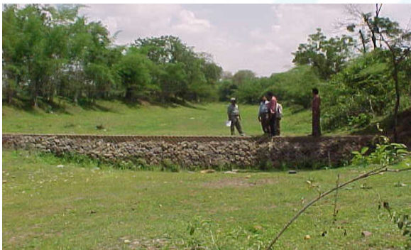
Figure 3.5 (c): Water harvesting gabion
