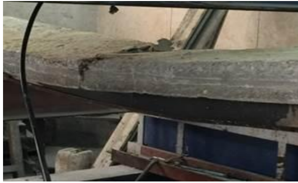
Figure 5.b: Cracks appeared in the surface of the concrete slab (A-4)
