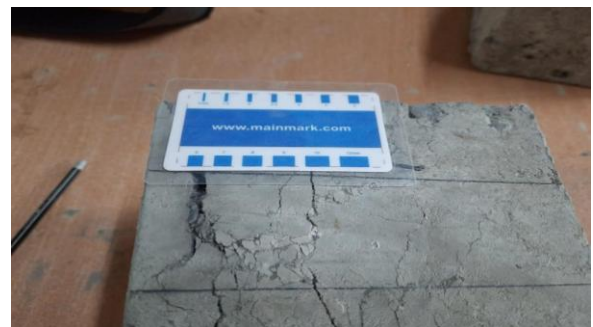
Chart 8: Measuring CMOD using Crack Width Comparator
