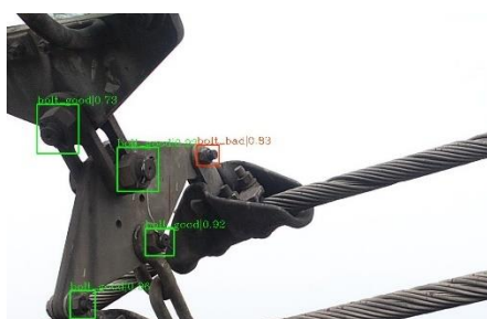
Figure 1: Bolts detection result of an inspection image
