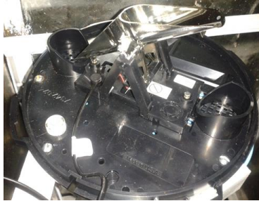
Figure 4: Interior of the rain gauge
