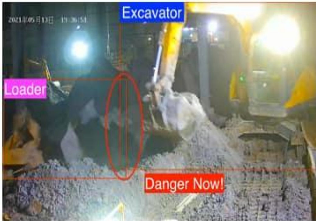
Figure 15: The autonomous excavator and loader potential. (Zhang & Zhang, 2021, p.52)
