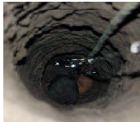
Figure 1: Image of a baby fell into borehole
