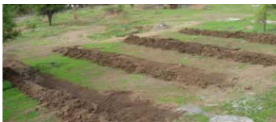
Figure 3: Continuous Contour Trenches
