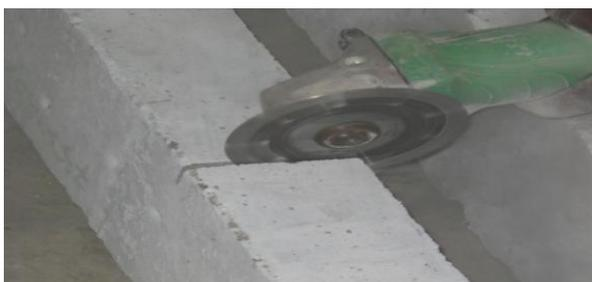
**Figure 3:** Cutting a Beam with Marble Cutter
