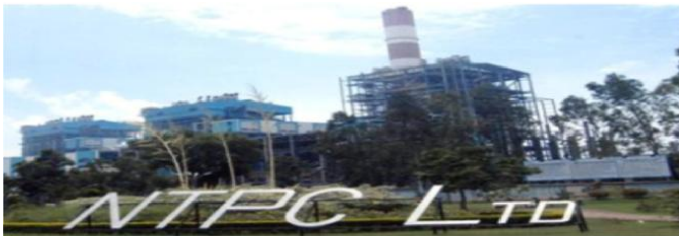
[Power generation from NTPC LTD]
