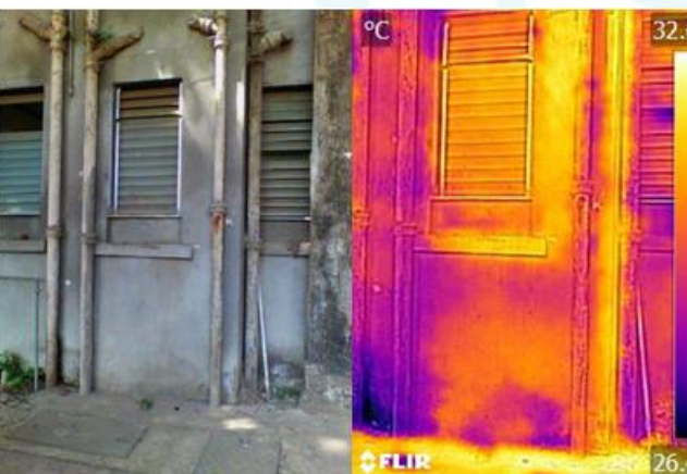
Figure 6: Behind Computer Department Toilet
