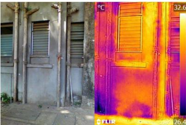
Figure 6: Behind Computer Department Toilet
