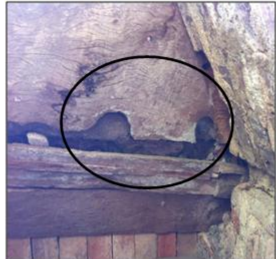
Figure 4: Timber decay at Saint Rose of Lima Parish Church
