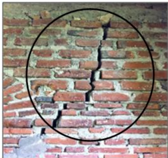
Figure 3 (b): Cracks on the walls of San Pablo de Cabigan Parish Church
