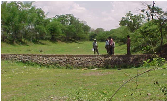
Figure 3.5 (c): Water harvesting gabion
