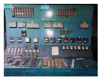
It is being difficult to maintain this DCS without spare support from OEM. There are several modules which will monitor and control important parameters like speed, power, position of control valve of the governor of TG-4 without which its generation can become zero MW. The capacity of TG-4 is 67.5 MW generating an income of Rs 130 lacs per day. By providing data of TG-4 on the system near Manager Intangible advantages are achieved for the Manager and the operator.
