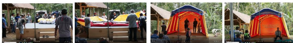
Figure 7: Inflatable Stage Roof Installation (6 minutes)
