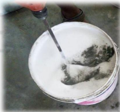
Figure 4: Mixing of Foaming Agent
