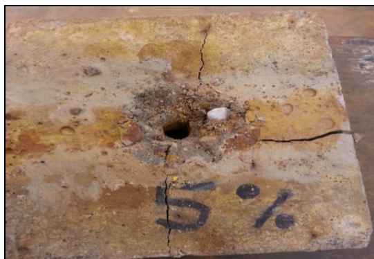
Figure 7: Concrete Specimens after Pull Out Test of 5% corrosion level
