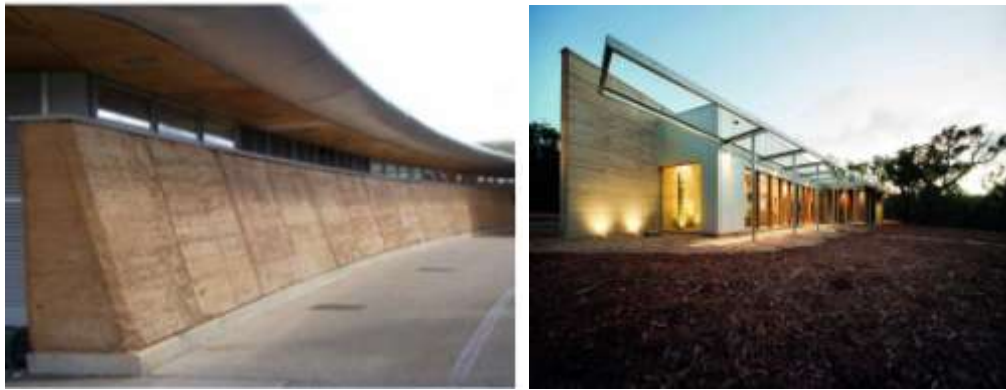
Figure 3: A rammed earth wall, fig.4 Hinderland house An Australia made of
