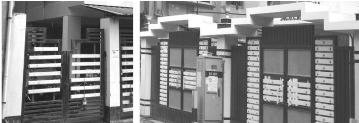
Figure 22 Boundary walls of new buildings. Source: Authors
