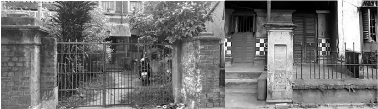
Figure 20 Boundary walls of old buildings. Source: Authors
