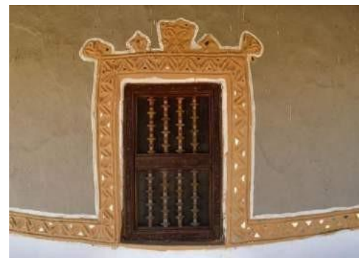
Figure 39. Timber framed window painted along the border.
