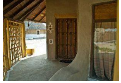
Figure 29. Clay wall Covered area.
