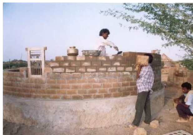
Figure 11. Clay Construction replaced with Concrete
