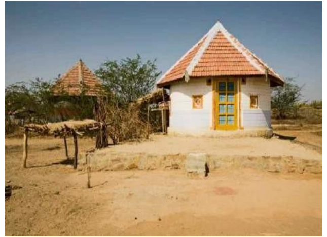
Figure 15. Raised plinth leading to bhunga with painted wooden door and windows.
