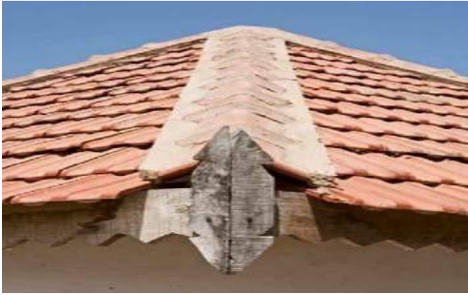
Figure 20. Detail of a construction joint of a hexagonal Mangalore tile roof.
