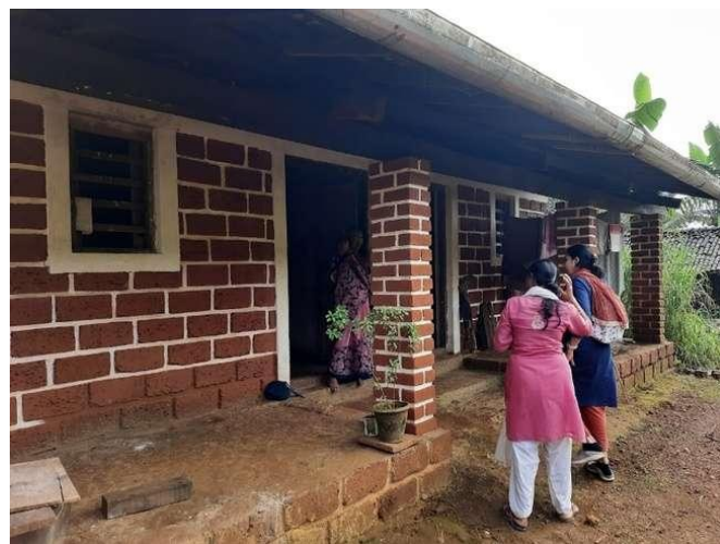
Figure 9 Recent houses made with laterite stones
