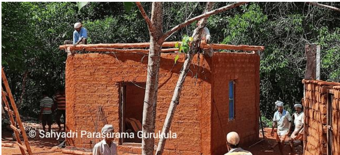
Figure 8 The Kutir/ residences made of locally sourced laterite stone
