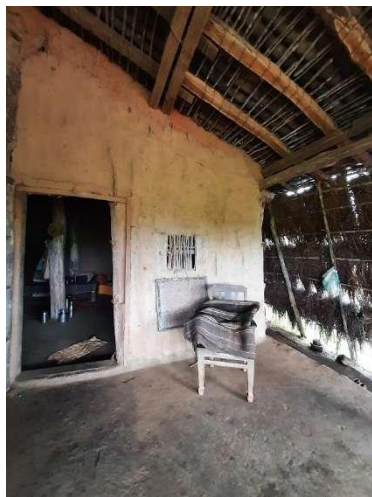
Figure 8 Mud house made with wattle daub walls
